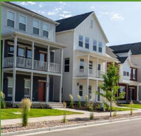
Image: Wilcox Farms Subdivision, Clearfield City
