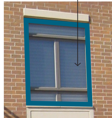
Measuring Transparency & Glazing on Each Story
